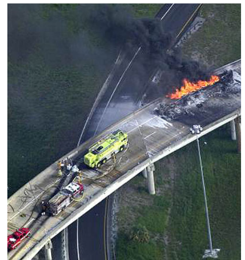
Orlando Florida Bridge Fire
