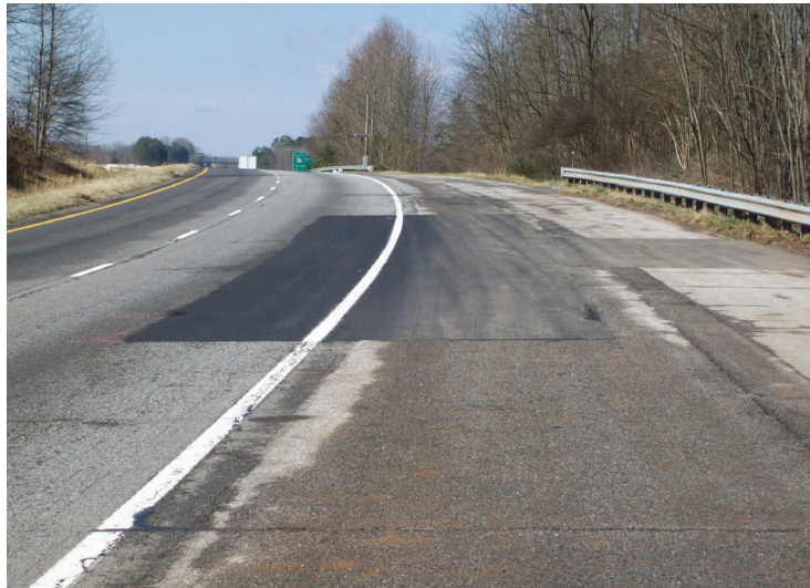
The completed repair to the sinkhole.
